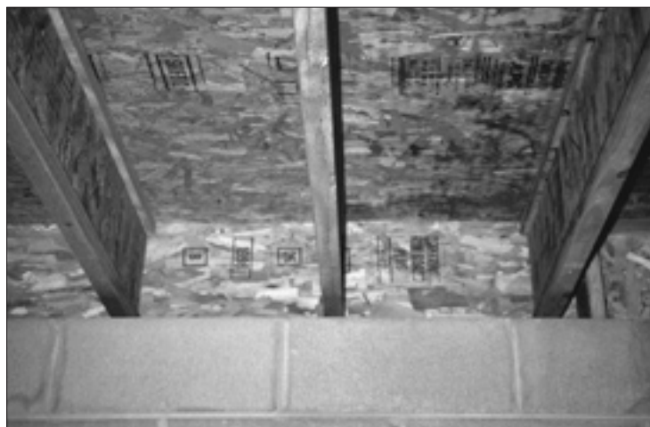
In this application, an engineered wood Rim Board is installed between the foundation sill plate and the floor under a wall section. The Rim Board matches the depth of the I-joists used in the floor framing.
