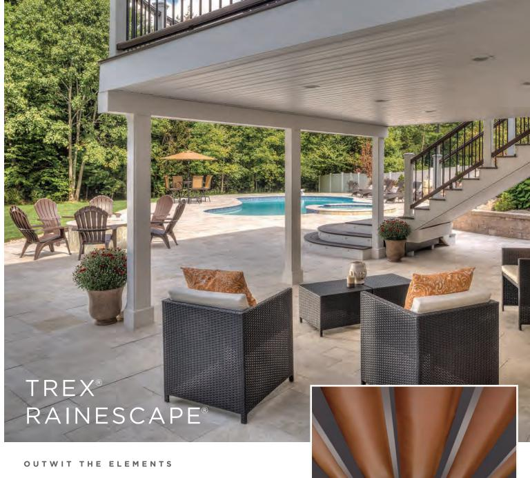
The unique Trex RainEscape under-deck drainage system keeps rain, spills and snow melt from dripping through the decking boards above, creating a dry room below.
